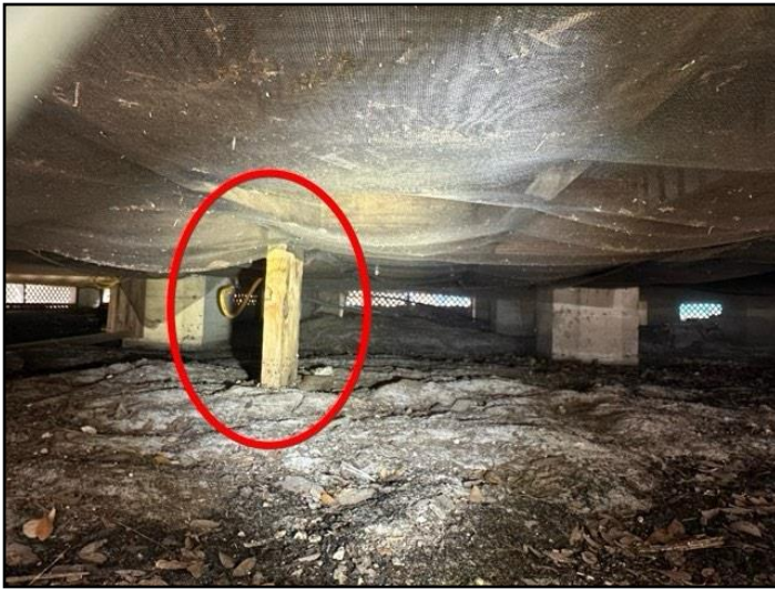
Multiple single board supports present
